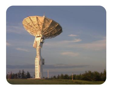
The ground station architecture makes it possible to operate the station locally via the user interface, or remotely via WAN. RF electronics are housed in the antenna structure to minimize losses.
